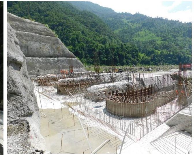
3. Concreting work at powerhouse foundation
