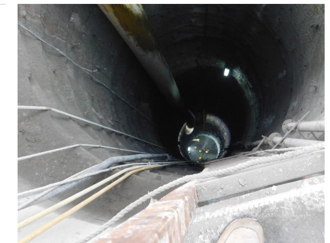
6. Vertical shaft excavation works
