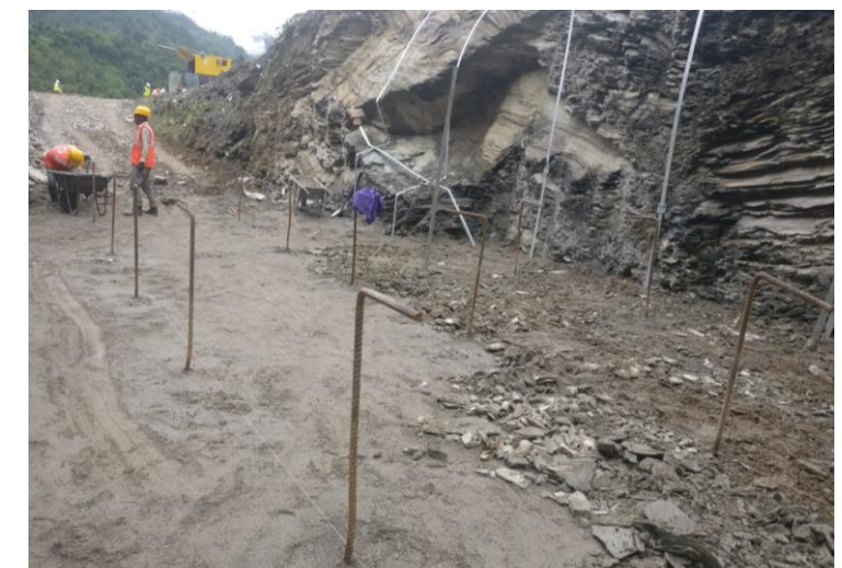
8. Laying of earth mat on powerhouse machine foundation
