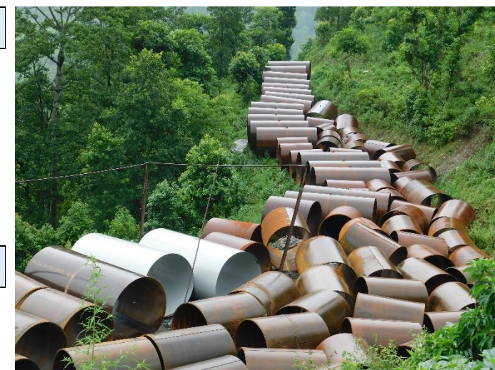
7. Penstock pipe after rolling at site
