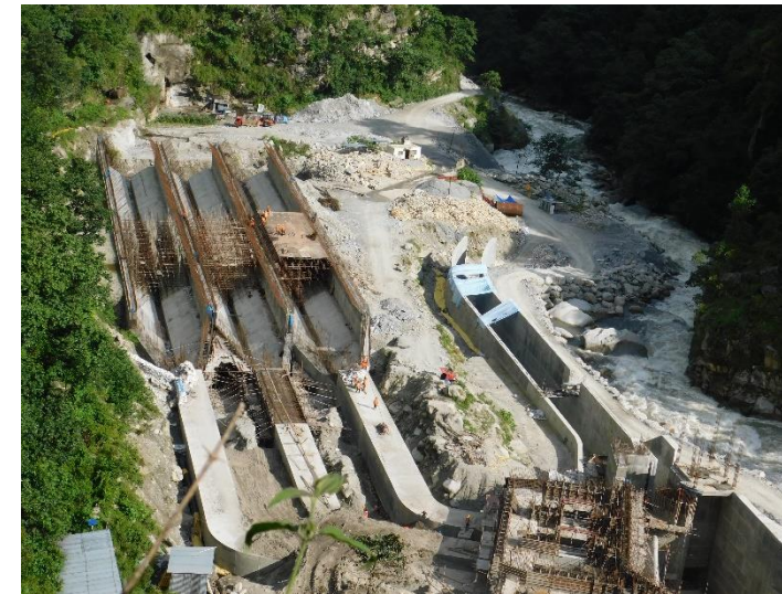
2. Gravel trap, sluiceway canal, approach culvert and settling basin.
