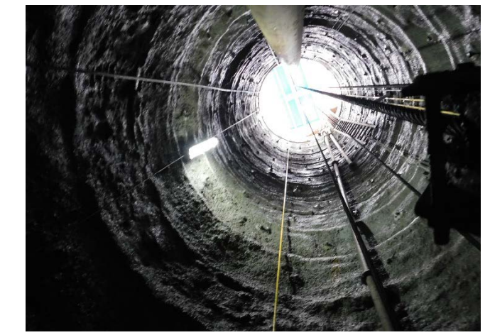
6. Vertical shaft excavation works
