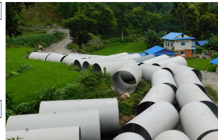
7. Penstock pipe storage after rolling and painting at the site
