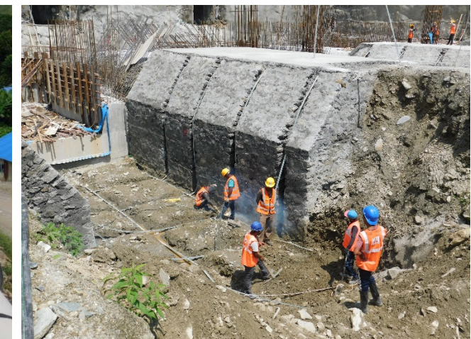
8. Laying of earth mat in powerhouse control building area
