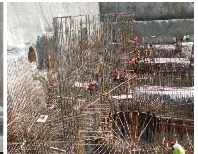
3. Concreting work at powerhouse foundation
