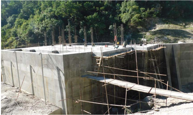
1. Headworks intake top slab concreting
