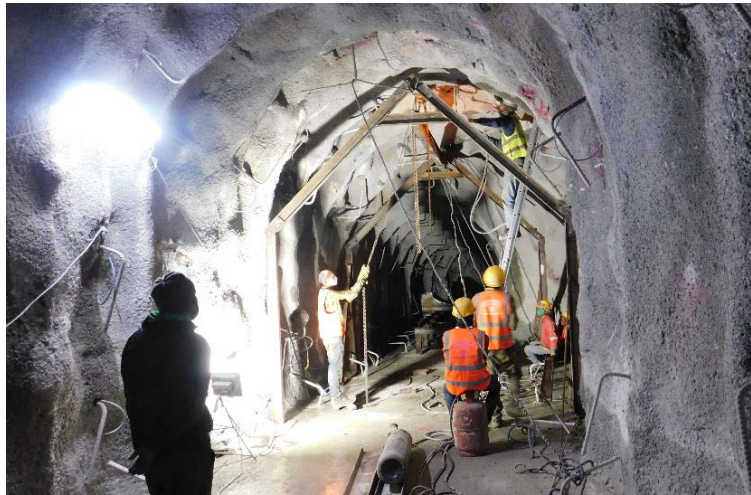
7. Preparation for penstock pipe fitting in bifurcation tunnel
