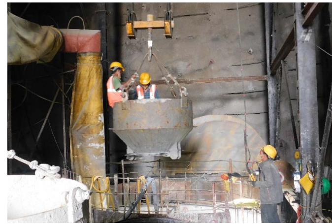
6. Winch Machine transporting the workforce to vertical shaft work place
