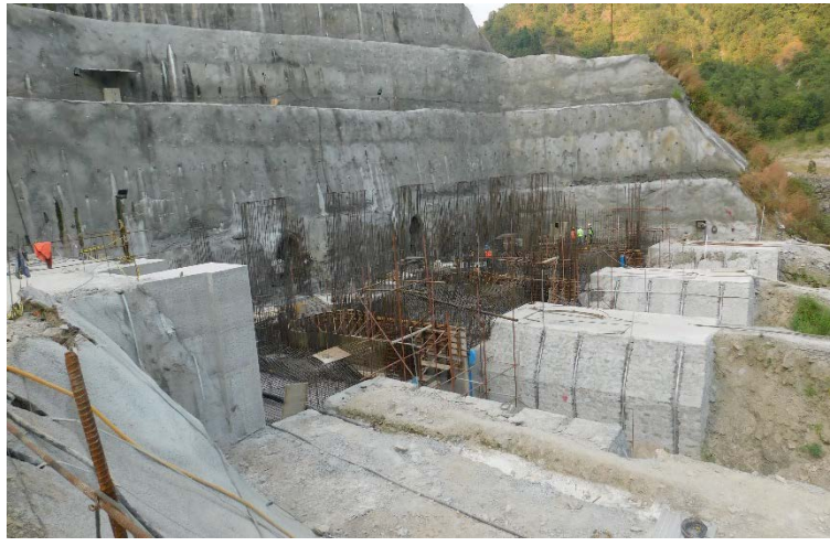
8. Laying of earth mat in powerhouse control building area
