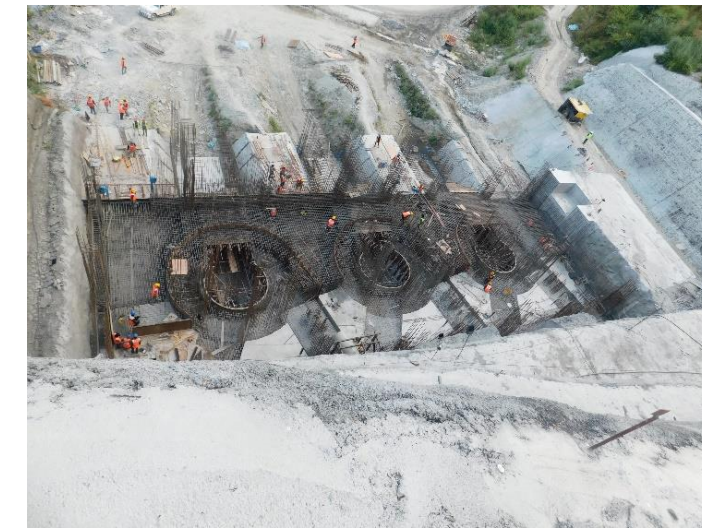
3. Machine foundation work at Powerhouse.
