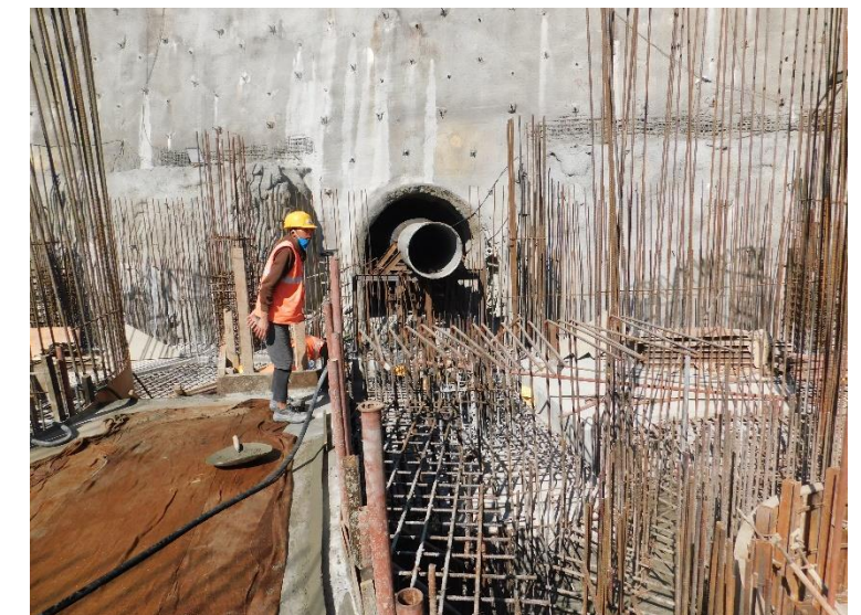
8. Penstock pipe fitted at one of the bifurcation unit.
