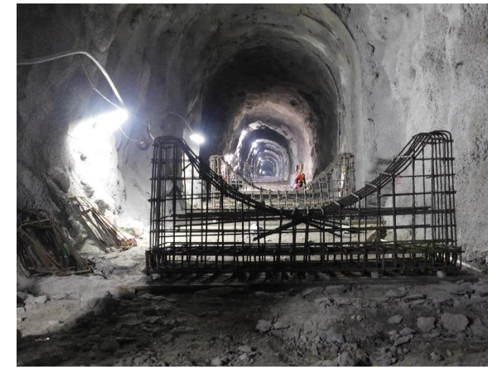
2. Saddle support preparation at penstock alignment
