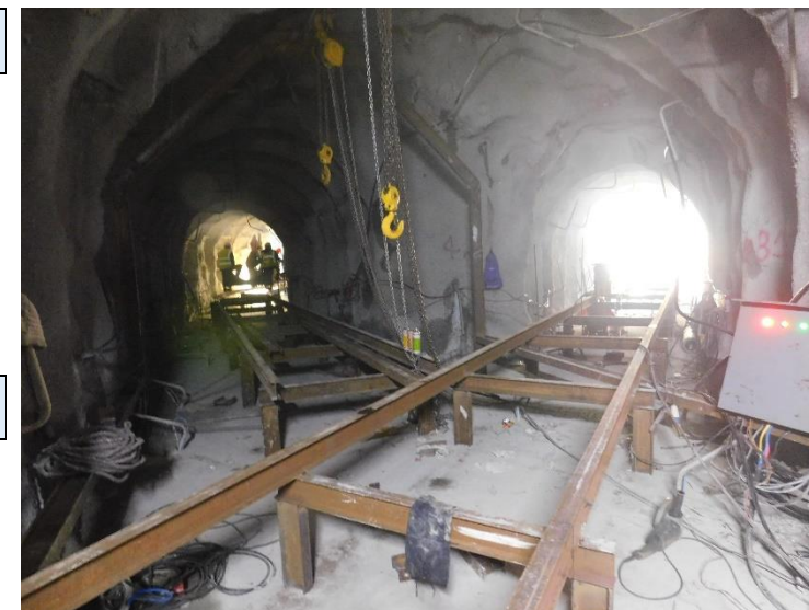
7. Preparation for penstock pipe fitting in bifurcation tunnel
