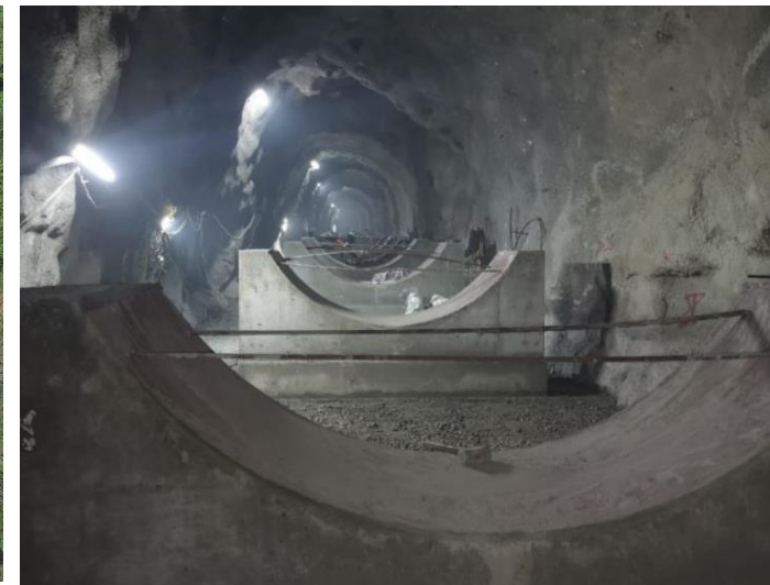
2. Saddle support at penstock alignment
