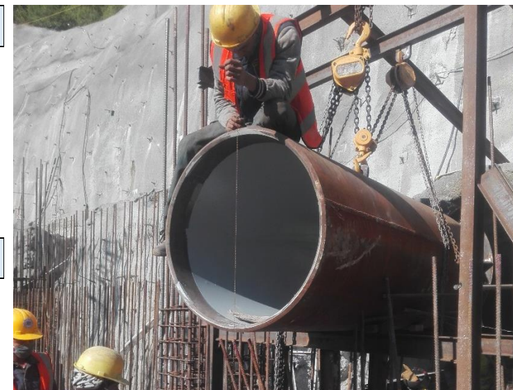
7. Penstock pipe fitting at powerhouse unit 1
