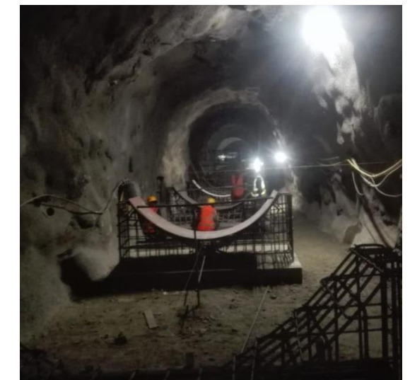
8. Saddle plate installing at saddle support.
