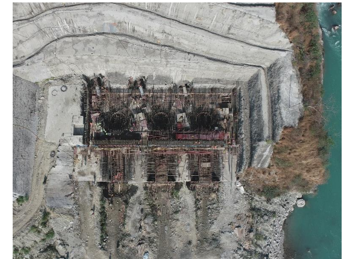
3. Machine foundation work at powerhouse.
