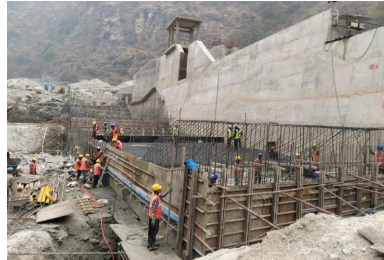
1. Weir and Stilling basin progress after 2 nd stage river diversion.
