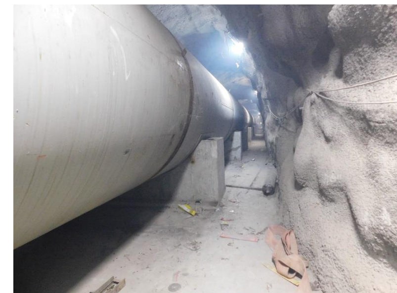
8. Penstock pipe installation at site
