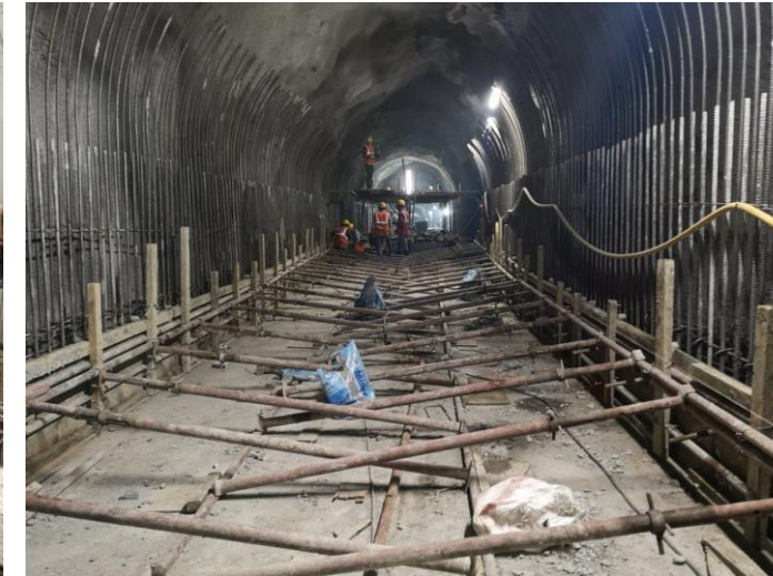
2. Concrete work at rock trap (Inside the tunnel).
