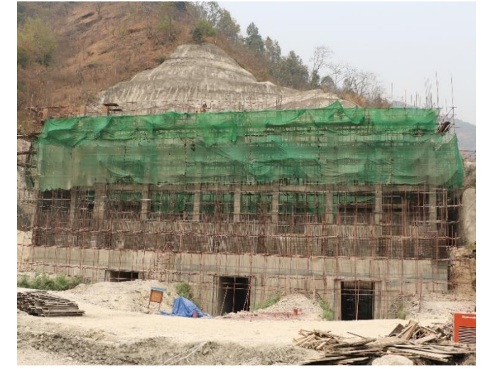
3. Powerhouse concrete works on progress.
