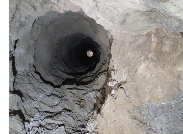
6. Ventilation shaft for surge tunnel break through
