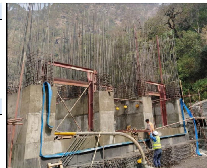
7. Outlet gate embedded part installation at Headpond.
