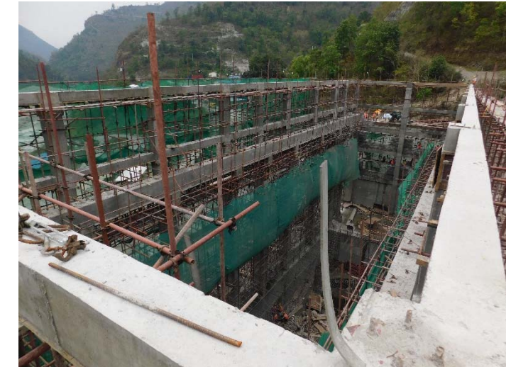
3. Powerhouse works on progress.
