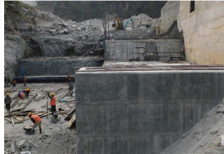
1. Weir and Stilling basin progress after 2 nd stage river diversion.
