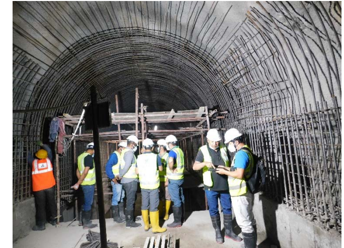
6. Technical team at Rock trap
