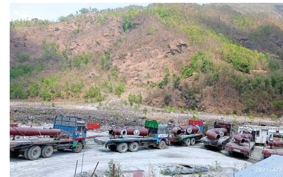
8. Electromechanical parts delivered to site
