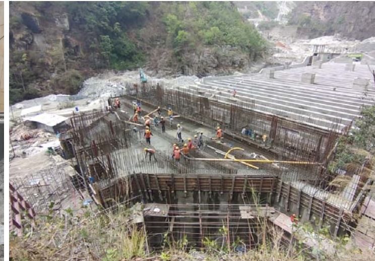
2. Settling basin and headpond nearly at completion phase
