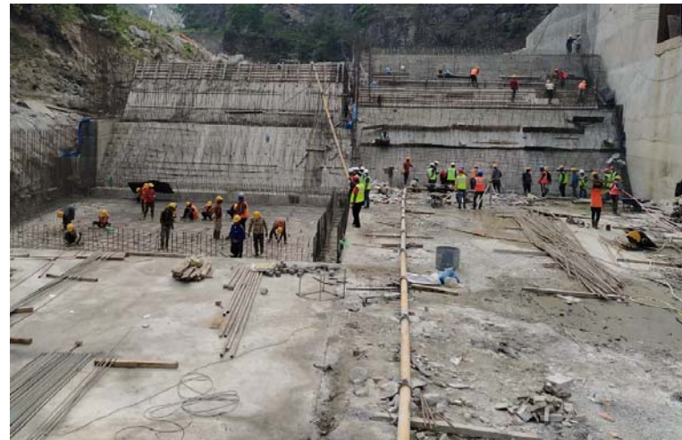
1. Weir and Stilling basin progress after 2 nd stage river diversion.
