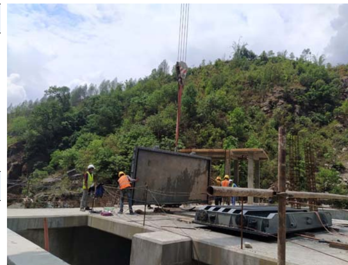
7. Installation of Intake Gate
