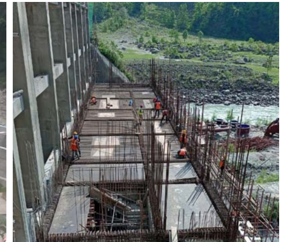
3. Control Building work at Powerhouse area.
