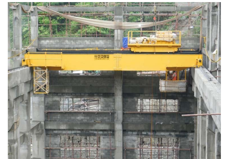
8. EOT crane installation at Powerhouse
