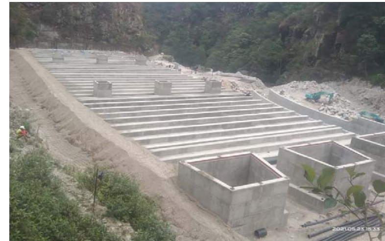
2. Settling basin view.
