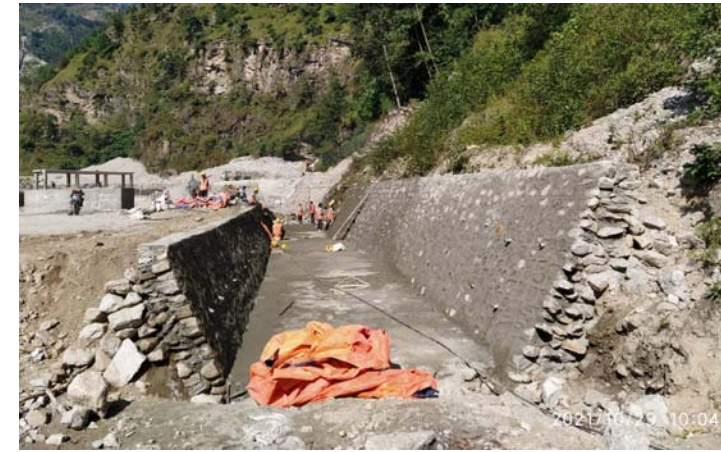
2. Surface drainage work at headworks area
