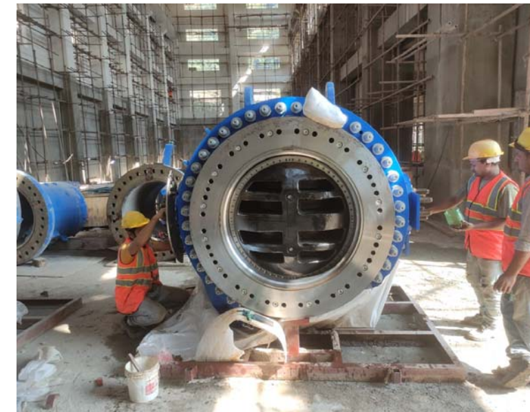
7. MIV ready for installation
