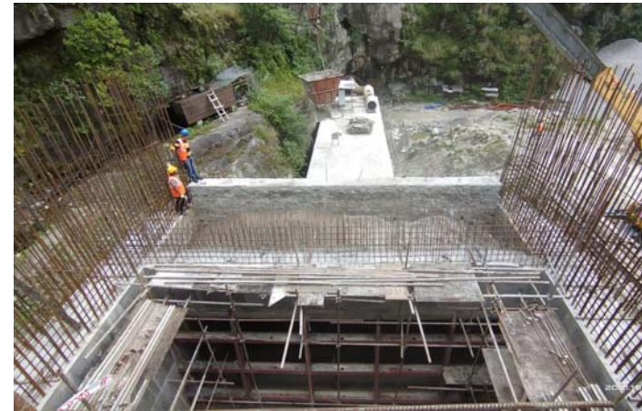
1. Headpond and Headrace culvert
