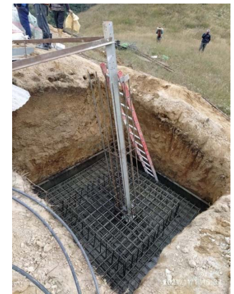
6. Transmission line tower foundation work
