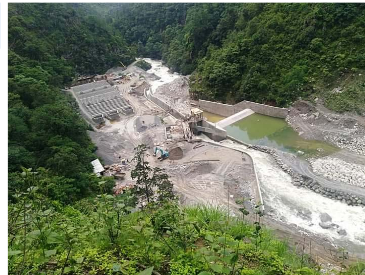
1. Headworks overall view.
