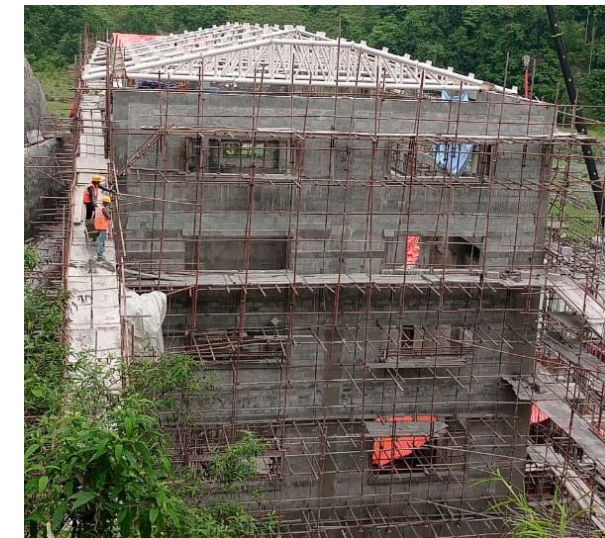
3. Roof truss work at Powerhouse
