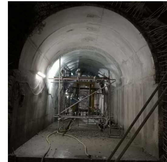
6. Concreting work at tunnel
