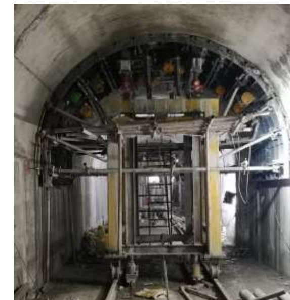
5. Surge tunnel permanent support work on progress.
