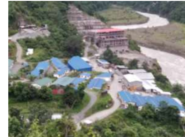
3. Progress at Powerhouse
