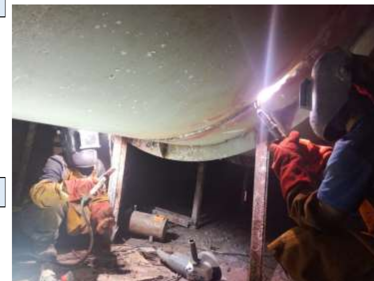
6. Penstock pipe welding on progress
