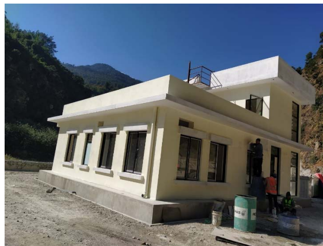
Figure 4. Painting work at control building of headworks
