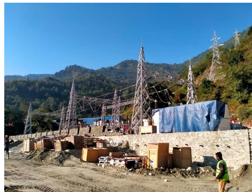
Figure 7. Switchyard and Transmission line work progress
