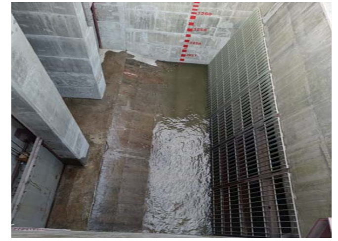
Figure 3. Water at headpond during water filling
