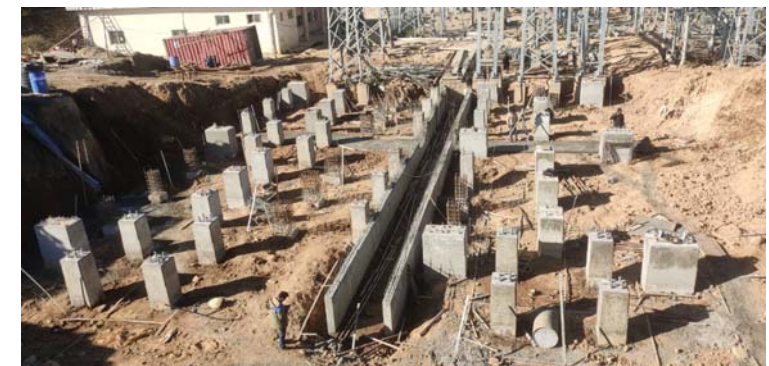
6. Foundation and cable trench work at interconnection bay, Tingla
