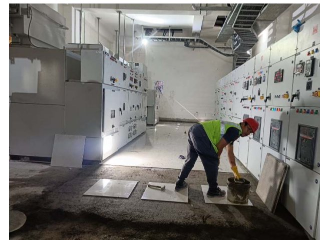
Figure 5. Tile work at Switchgear room
