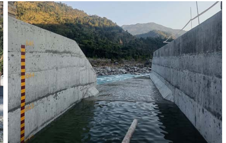
Figure 3. Dewatering from tailrace during testing
