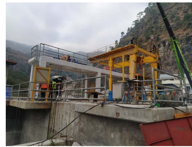
Figure 5. TRCM installation at intake area
