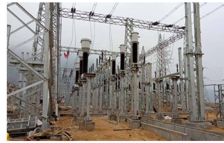
6. EM work progress at interconnection bay, Tingla
