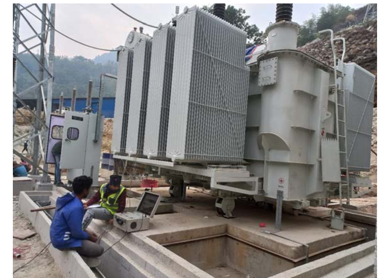
Figure 8. Testing of Transformer
