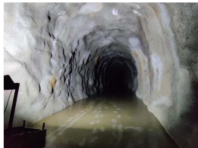
Figure 4. Dewatering of headrace tunnel
