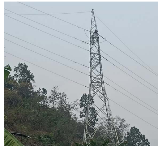
Figure 5. Conductor laying
