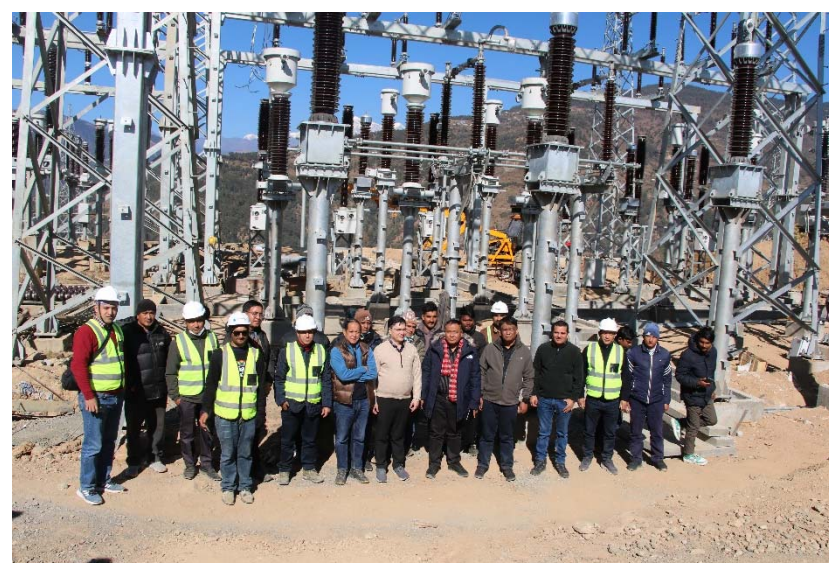
Figure 7. NEA MD and team at Lamanne Substation for monitoring the work progress
