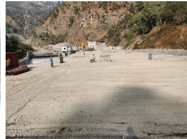
2. Settling basin area
