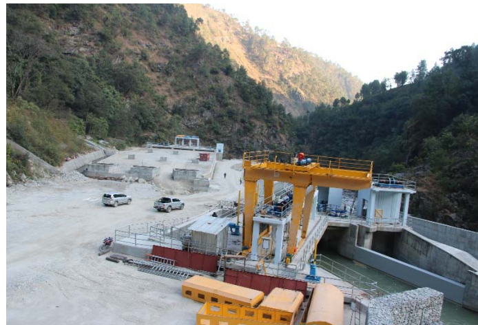
Figure 4. TRCM installation at intake area
